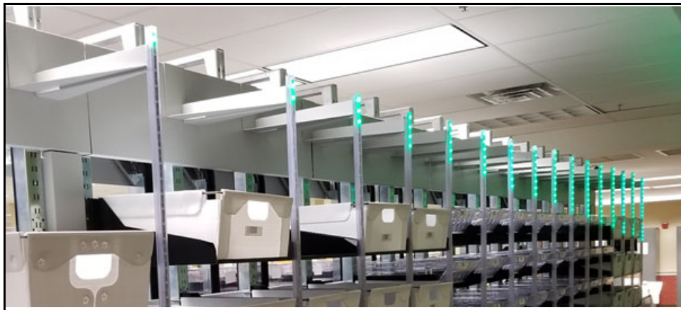
Figure 3-5: Vertical LED Strips
