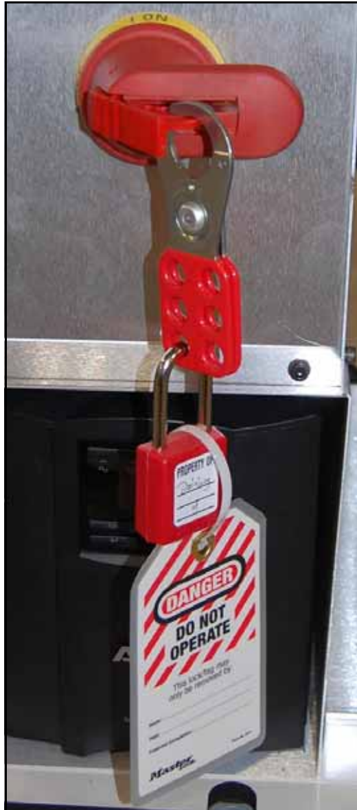
Figure 2-15: Lockout Tab with Hasp, Padlock and Tag
