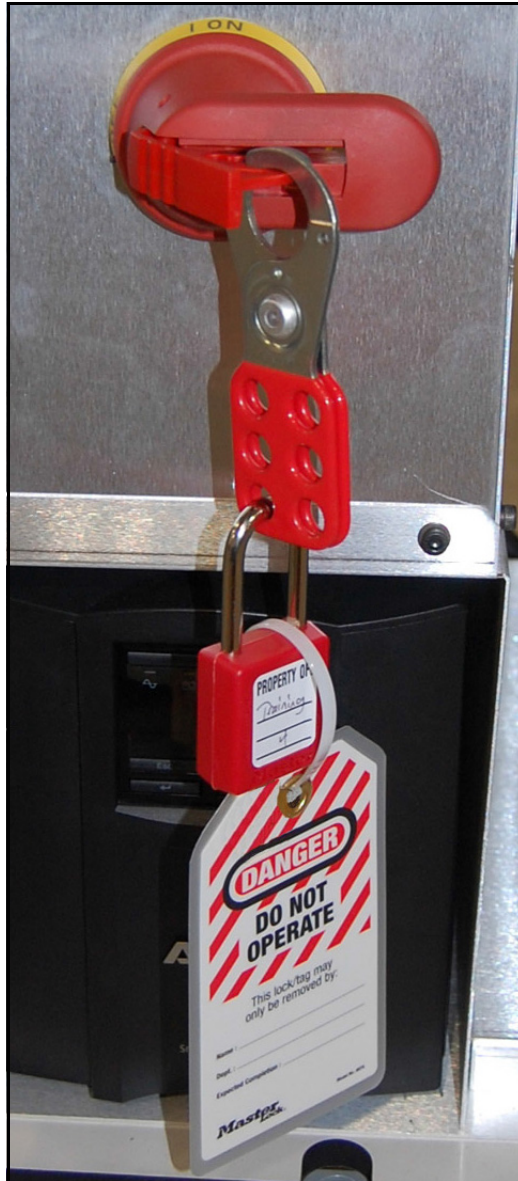
Figure 2-16: Lockout tab with hasp, padlock and tag
