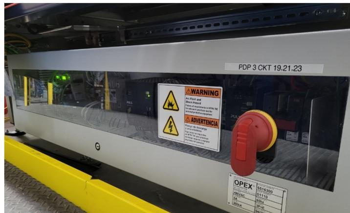
**Figure 3-15: Main power switch on workstation MCP**
